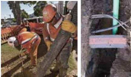
**Hydroexcavation allows you to safely dig without fear of hitting underground pipes or wires while keeping mess and scarring to a minimum.**
