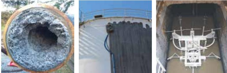
***Our UHP water jetting resources include robotic units that give us capability to tackle the toughest jobs, such as clearing this heavily scaled 400m pipe (left), large scale tank surface preparation (centre) and sewer corrosion removal (right)***
